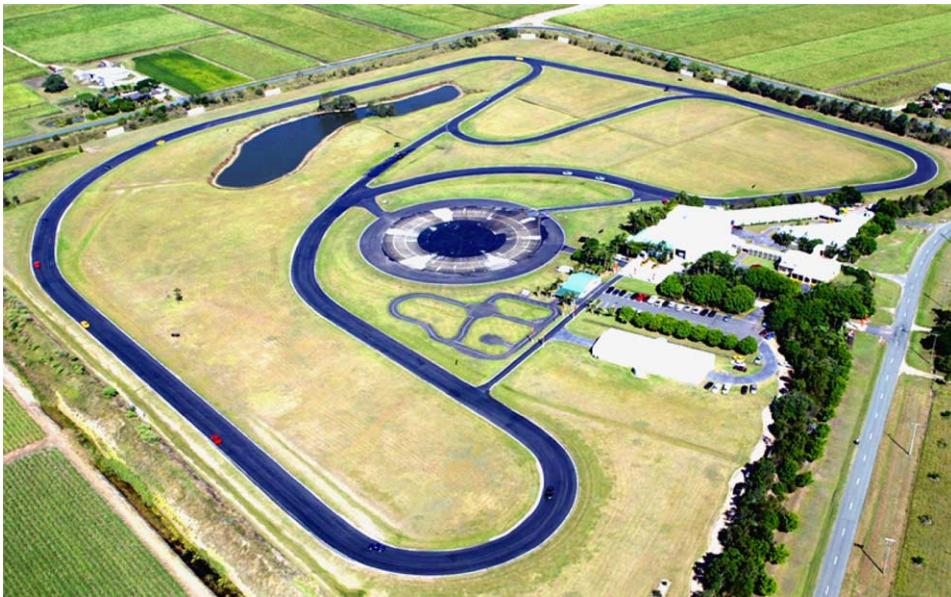
Fig. 1. Aerial view of the Holden Performance Driving Centre (HPDC, Queensland, Australia).
